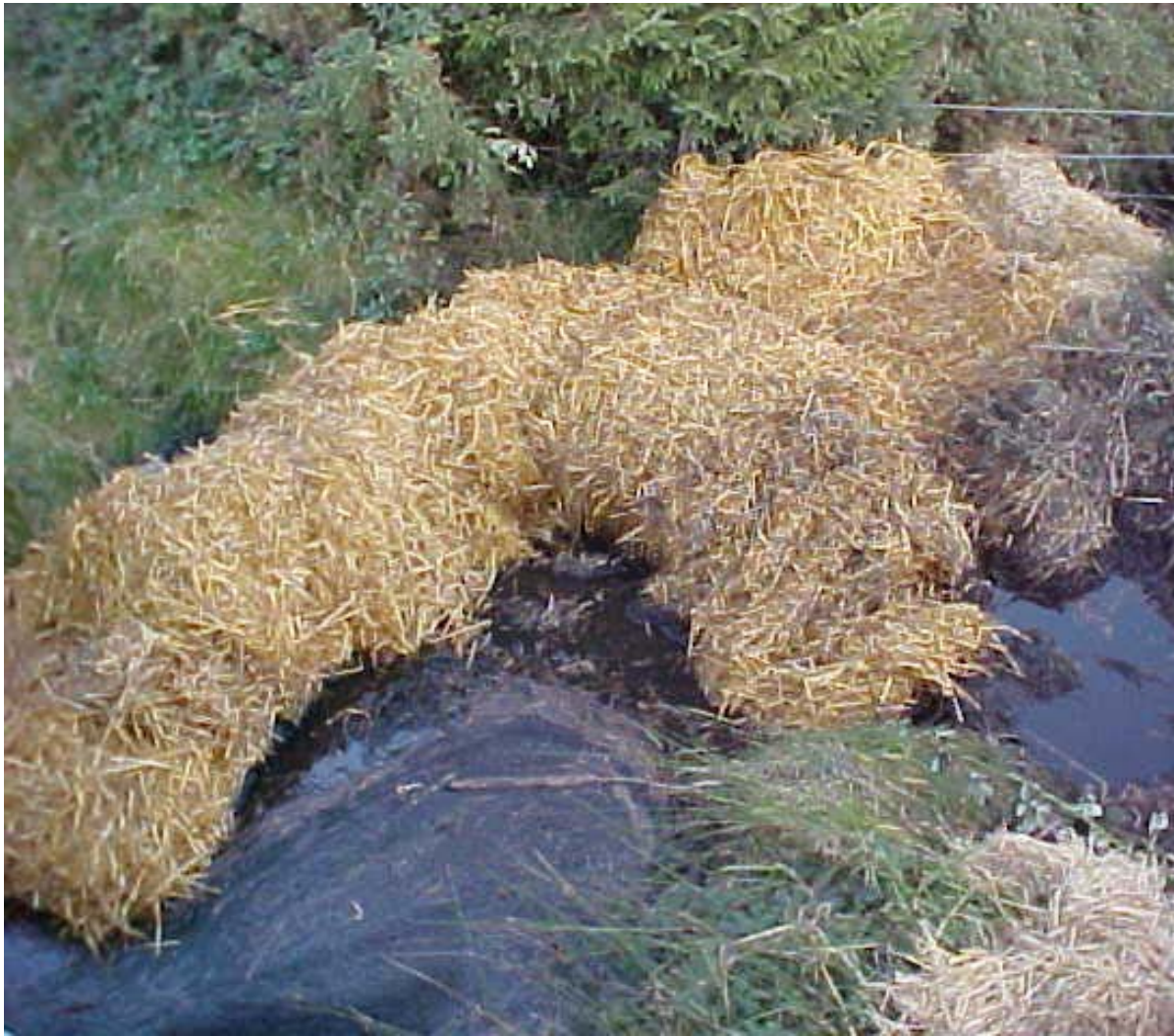
Plate 11.3 Straw bale filter on wind farm site
