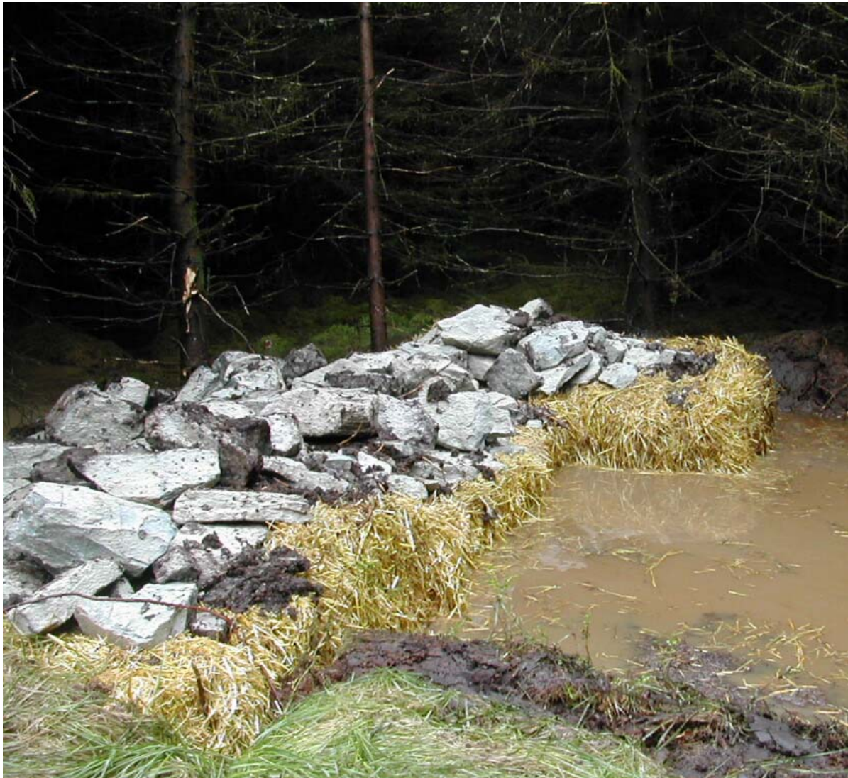
Plate 11.4 Silt trap installed at exits from wind farm site
