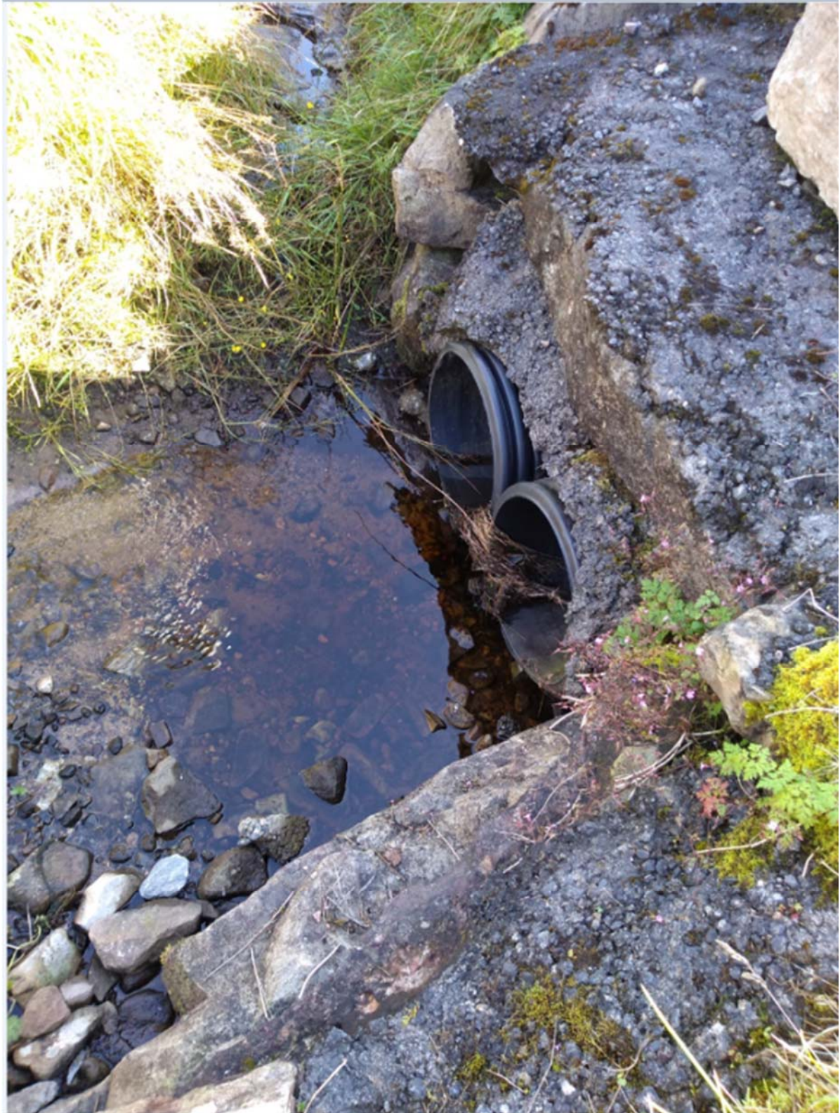
Plate 11.7 Twin 600 mm pipes at crossing near T35
