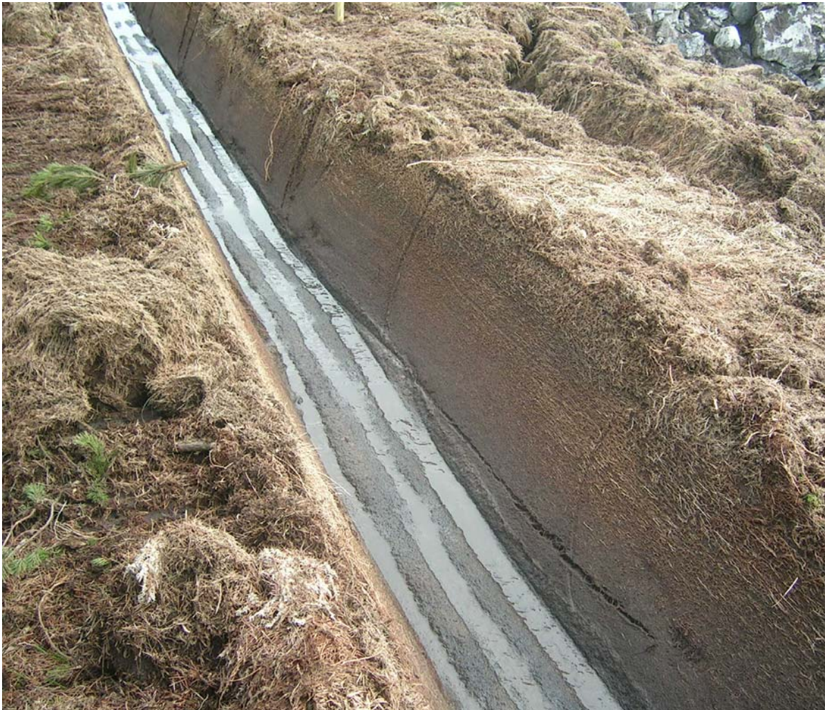
Plate 11.6 Typical drain installed during wind farm construction
